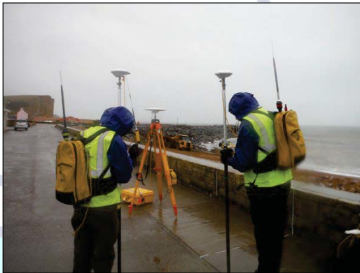
Figure 4 The SWCM team surveying Porlock.
