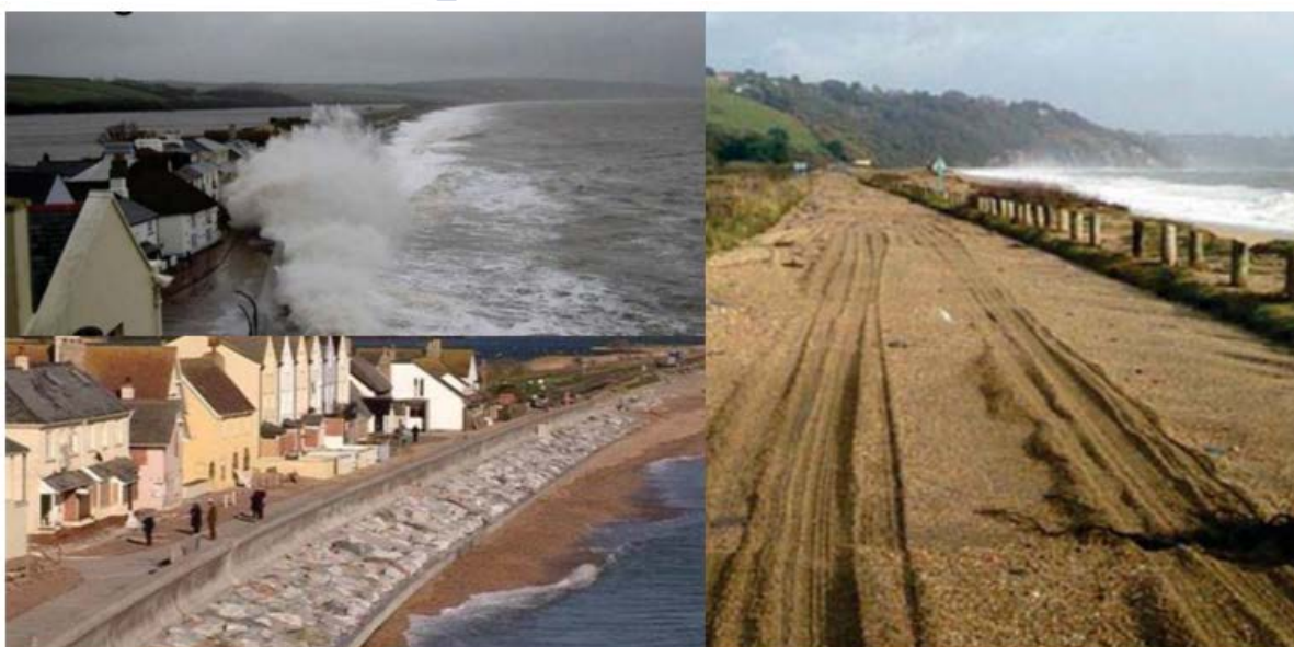
Figure 7 2013/2014 Storm events. Waves crashing over the sea defence, uncovering of the bottom of the sea defence at the souther end of Slapton Sands and the road at the northern end covered in shingle
