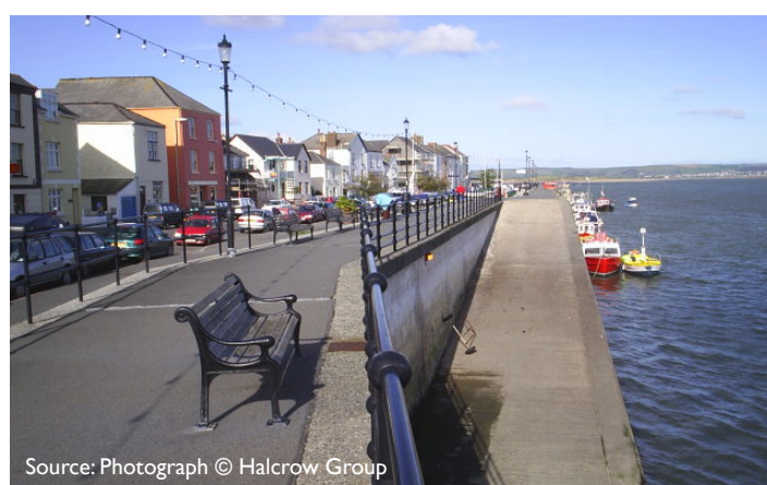
Source: Photograph © Halcrow Group
