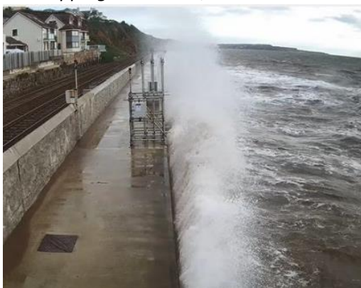
Overtopping at Dawlish, 7 th March 2022
